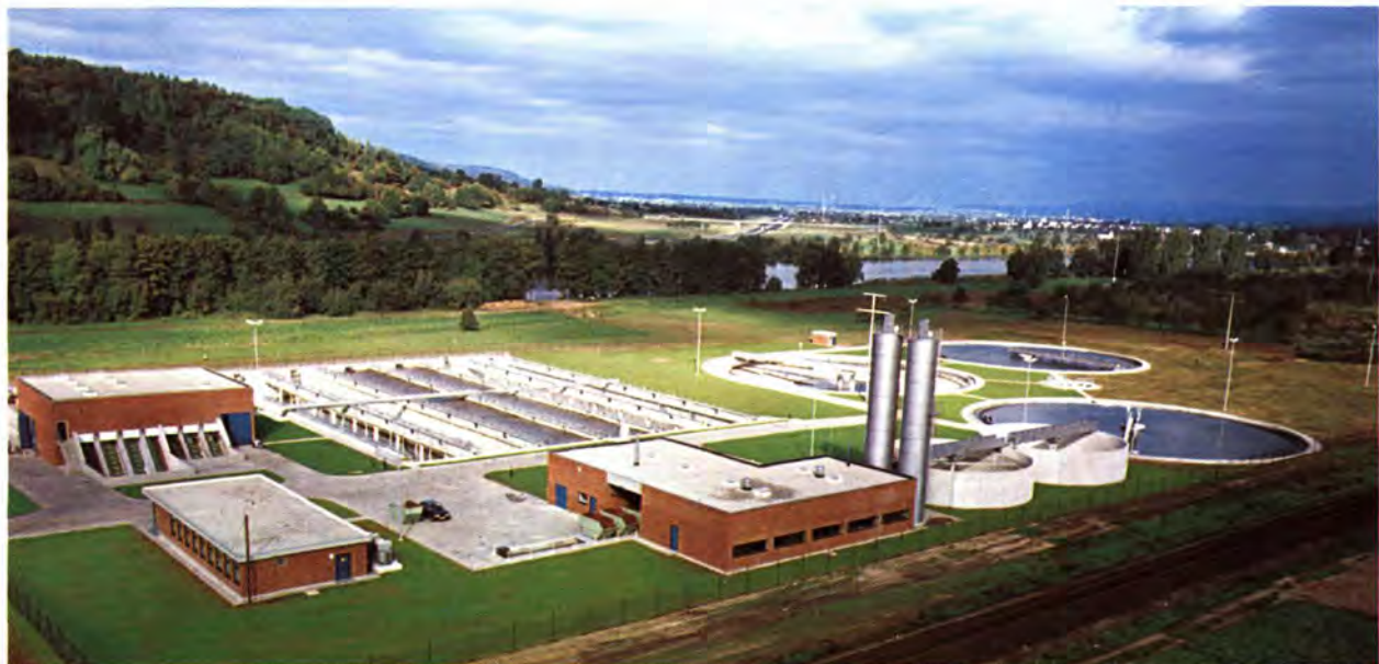
The biochemical purification plant of Enka Glanzstoff's fiber complex at Obernburg (West Germany) came on stream in 1976. It can treat up to 2,500 m 3 /h of industrial effluent, plus 500 m 3 /h
