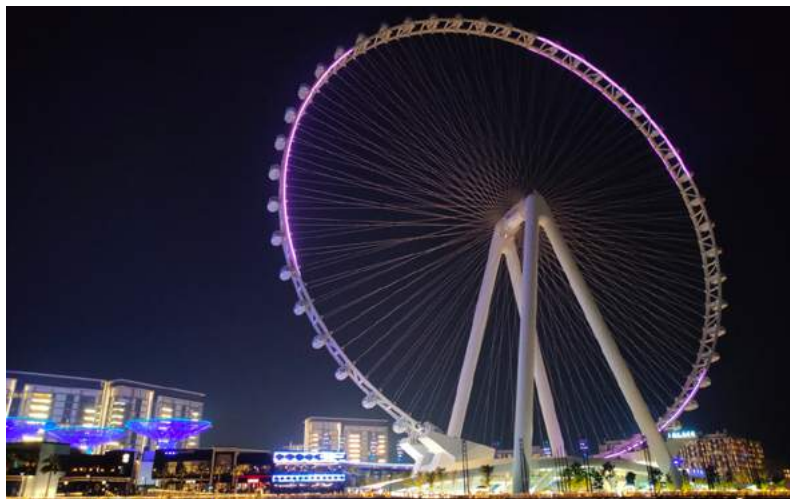
This is the hugely impressive Dubai Eye, the world's highest and largest Ferris wheel, which was opened to visitors in late 2021. Measuring a dizzying 250 meters and featuring more than 9,000 tons of steel, we were sole supplier of protective coatings for the massive structure. It means we've now coated four of the world's most iconic observation wheels, the others being the London Eye, Melbourne Star Observation Wheel and Singapore Flyer.
