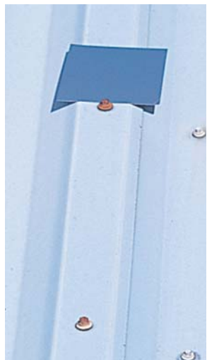
No comparison Close-up of original paint chip of competitive SMP coating on faded metal roofing, after ten years in Ohio weather.
