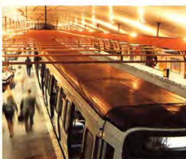
Twaron ® aramid fiber has applications in numerous fields. Shown here is its use as tensioning member in the roof of a Paris subway station.
