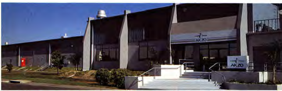
In January 1989 the new manufacturing complex in Orange, California, United States, was inaugurated. It is the center of all our coatings activities on the west coast.
