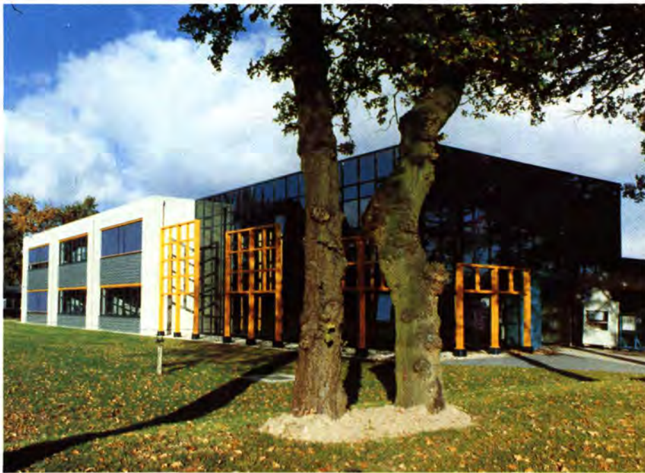
Up to 400 young people from Akzo plants and other companies can be taught engineering skills in the new technical training center in Emmen, the Netherlands.
