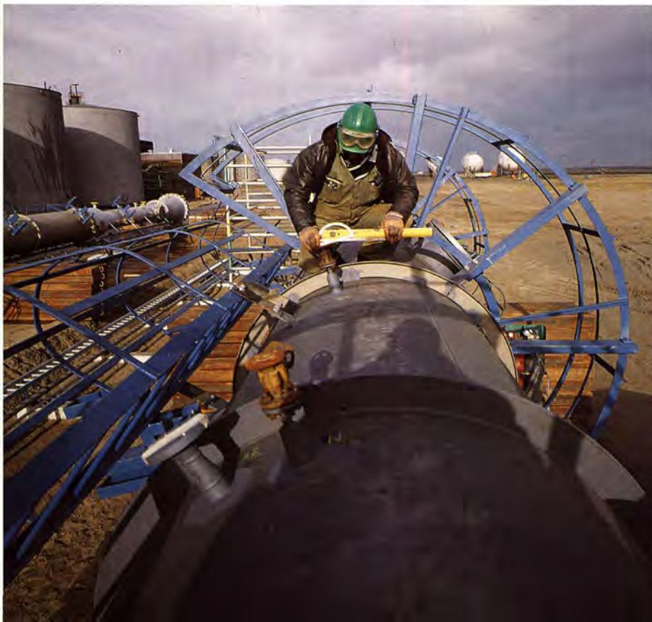
Detail of the DME plant under construction in Rotterdam, the Netherlands.
