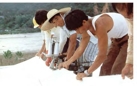
Geosynthetic materials for soil stabilization.
