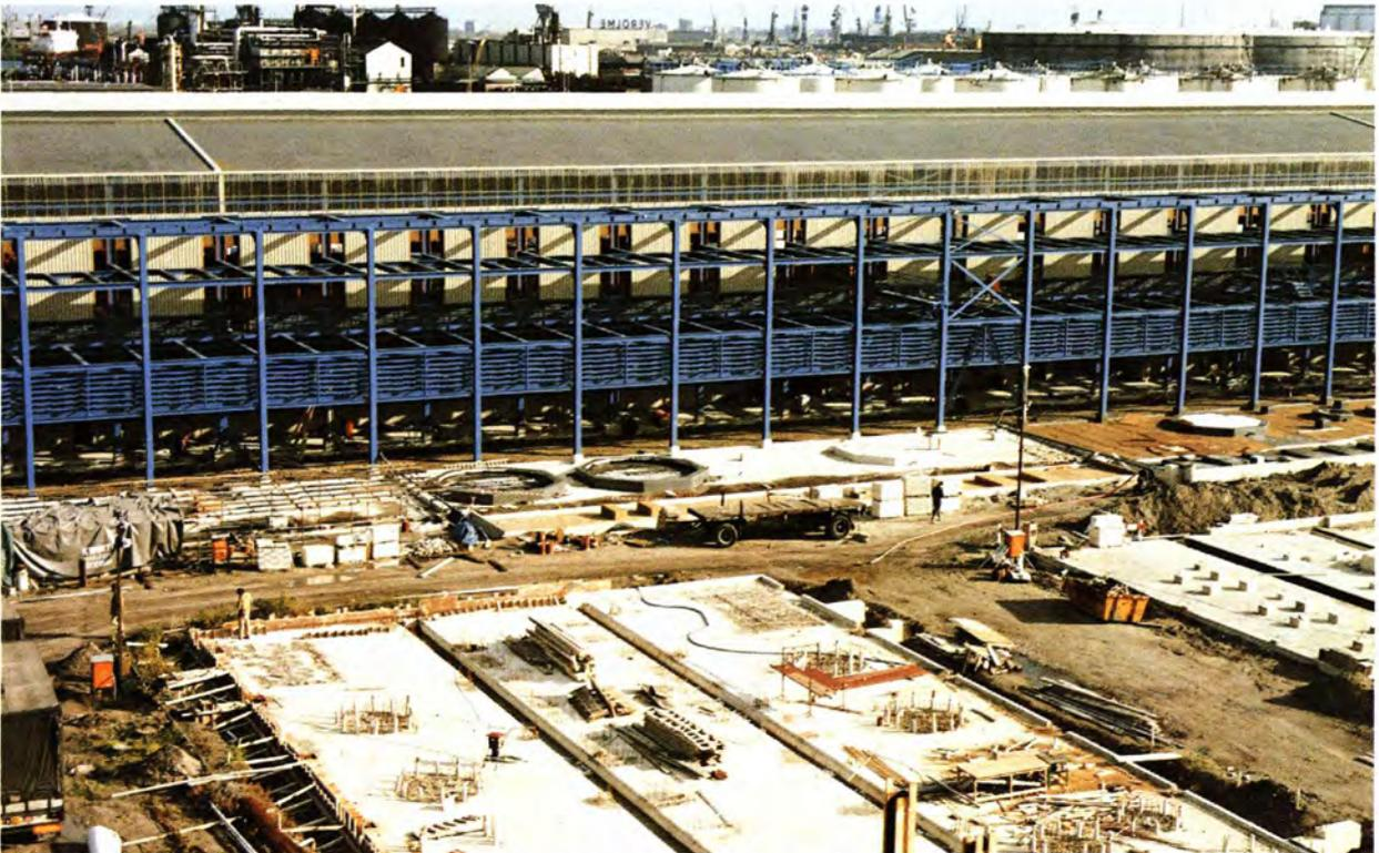
*Akzo Engineering designed the new Rotterdam electrolysis plant and will also supervise erection. The plant, scheduled for completion in early 1983, is to have an annual capacity of 250,000*
