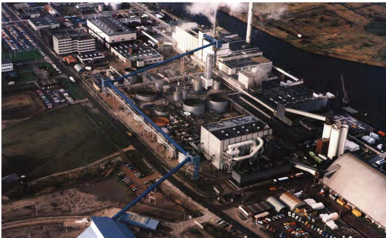
*The new, coal-fired, fluidized bed boiler at Hengelo, scheduled to be started up in the fall of 1986, permits efficient and environmentally clean energy production. In combustion, coal and lime are suspended on a column of air,*
