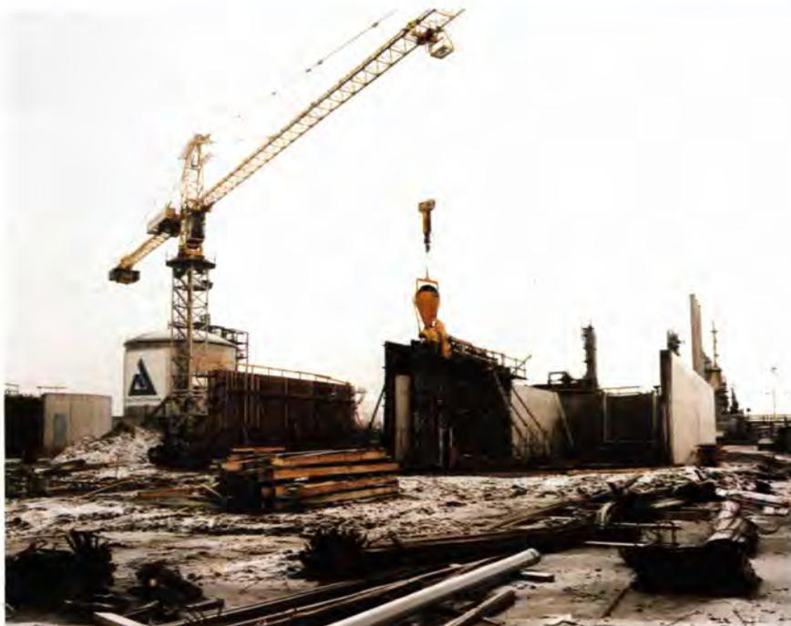
*This purification plant in the Rotterdam Botlek area will treat wastewaters of the crop protection chemicals and vinyl chloride monomer plants. In the biological purification stage, powdered activated carbon will be added to the pretreated effluent as an adsorbent. Past experience has shown this addition to be highly effective.*
