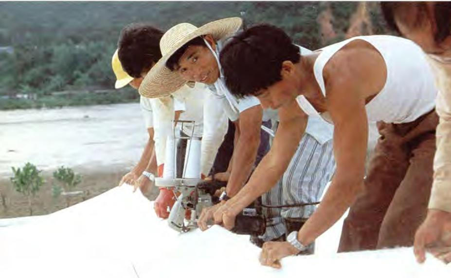
*Geosynthetic materials for soil stabilization.*
