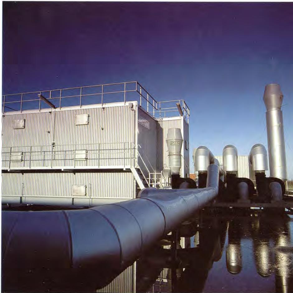
*New biofilter installed at the Sassenheim, the Netherlands, location absorbs the greater part of the hydrocarbon emissions passed through it.*
